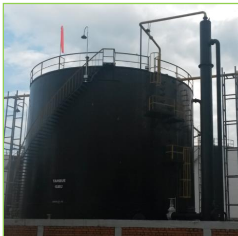
Figura No.24 Gun Barrel 1000-2 S-ABK 102
